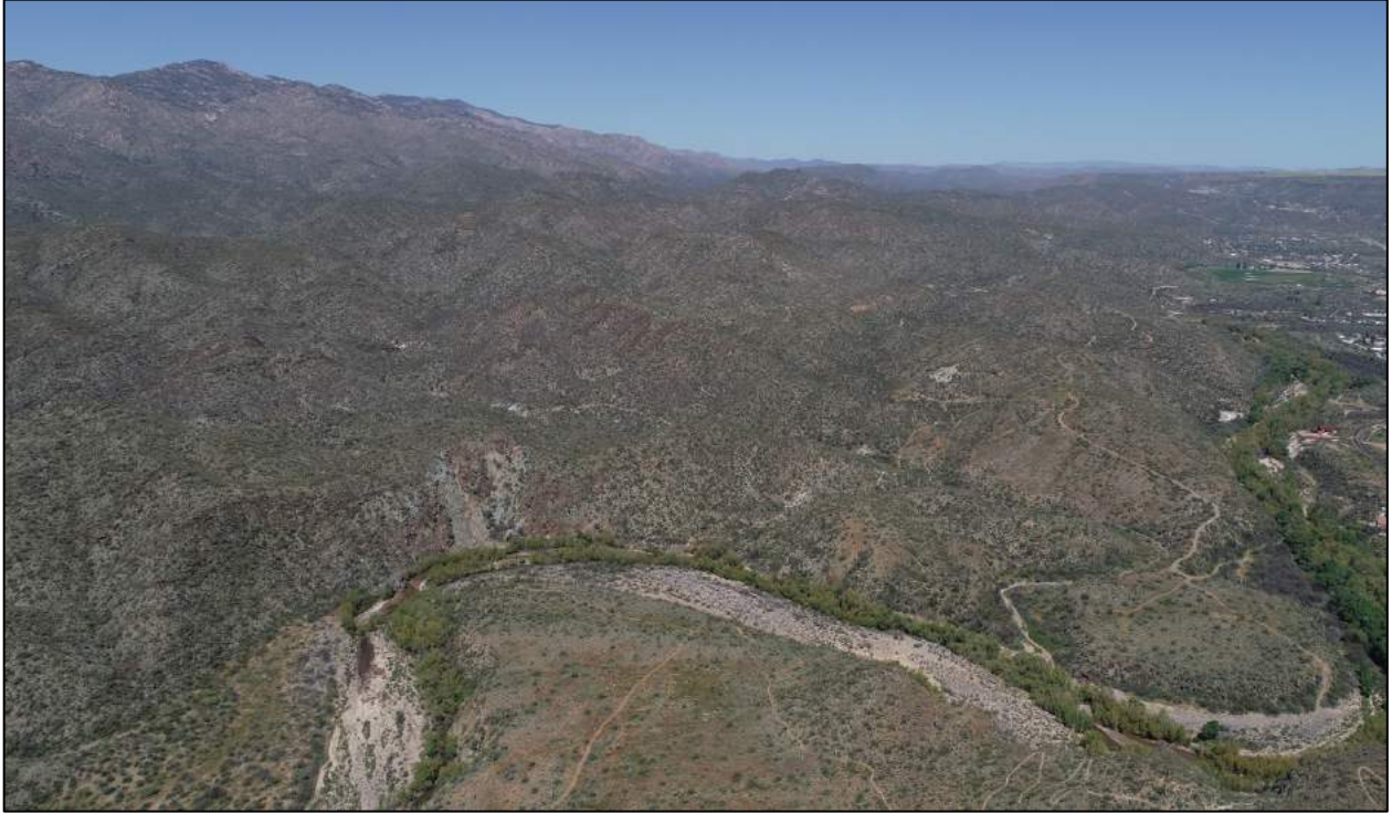
Figure 3. Aerial view of the project looking north.
